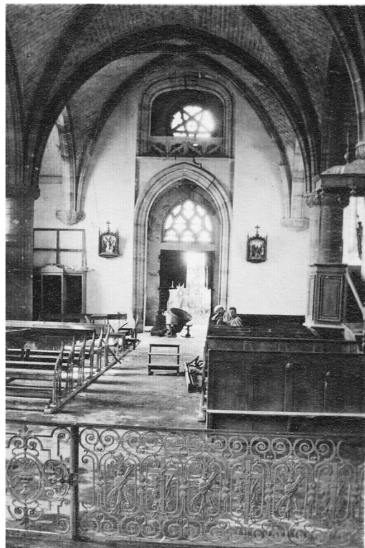
Villers aux Vents Church
